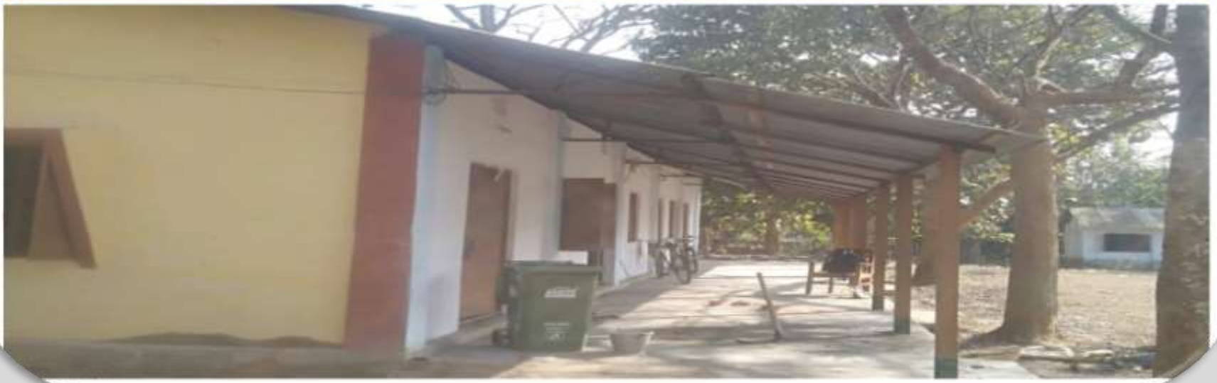
Maintatnance of Rajkang VC and Construction of Shilaphalakam
