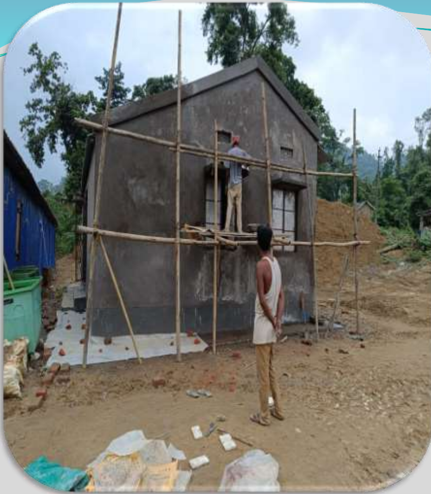
A photo of the New Anganwari Center during its work
