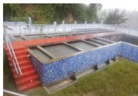
Horizontal Roughening Filter Cum Slow Sand Filter
